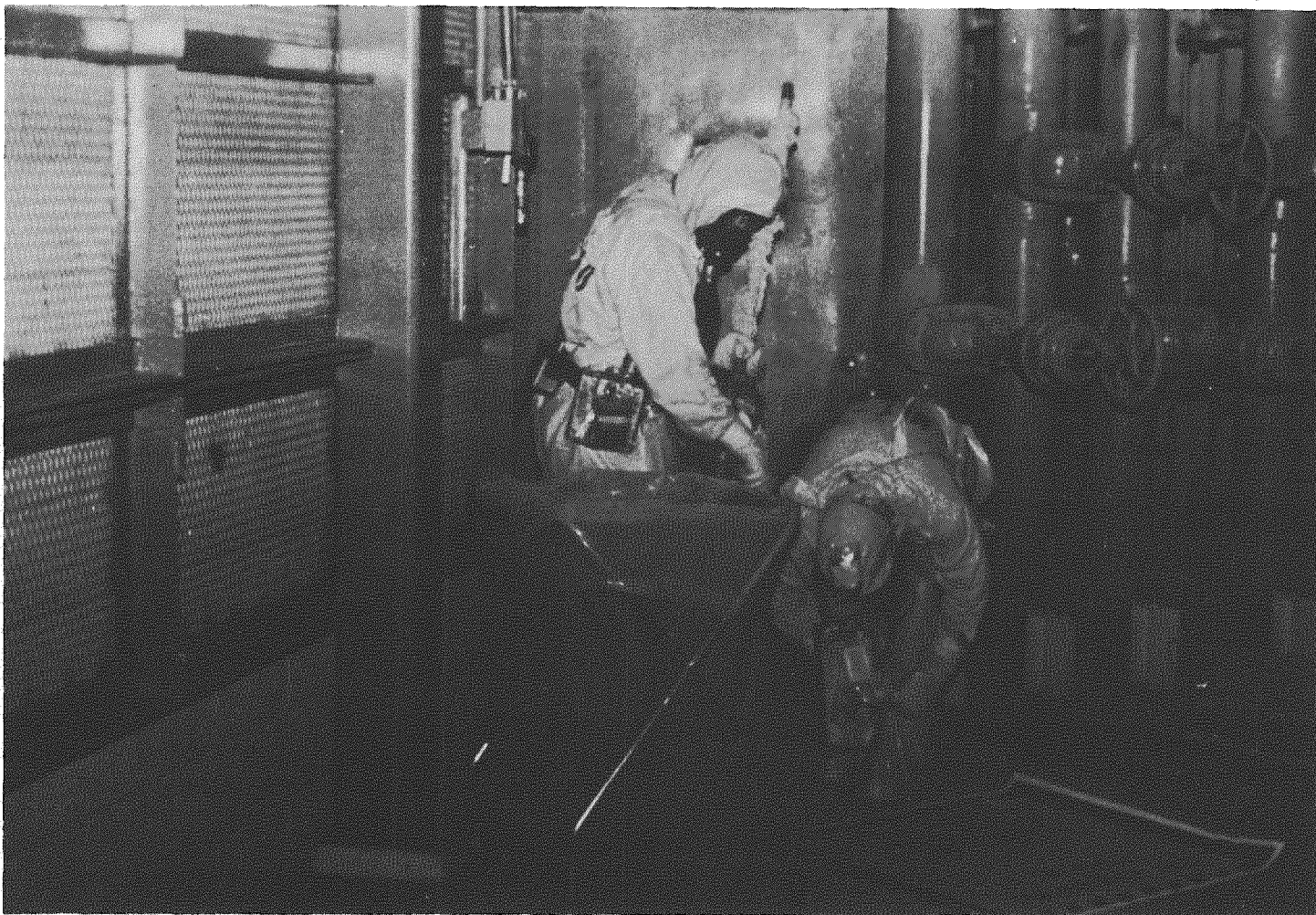
Technicians remove outer set of protective shoe covers at contamination control area on the 305-foot elevation. (TIO Photo Entry 11)
